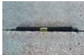
Concrete floor Location from Storage Areas
