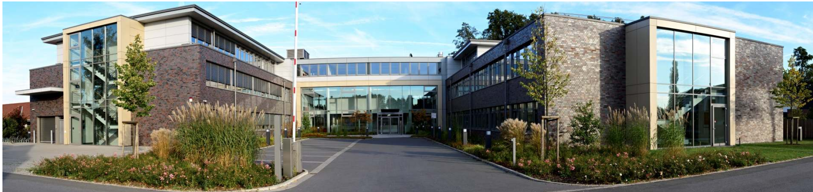
Beckhoff Corporate Headquarters and R&D Centre
